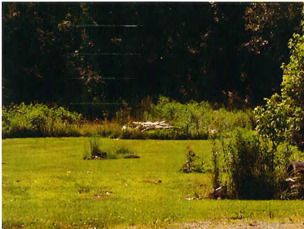
Date: 6/17/2014 Time: 10:06 a.m. Direction: east Photo by: M. Stevenson Exposure #: 004 Comments: construction demolition debris
